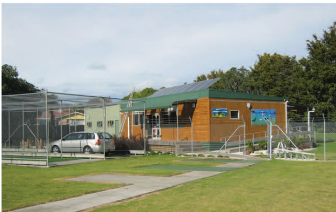
Photovoltaic panels at Whakatane Intermediate School with north facing orientation on a tilted frame. Note the south sloping roof angle
