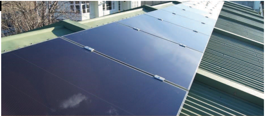
Thin-film silicon on glass used with the Lake Tekapo Schoolgen installation. Note the larger area of the panels to generate the same amount of electricity.
