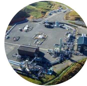
Creating fuel and plant flexibility
