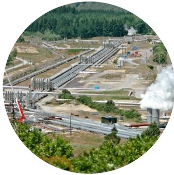
Considering PPA Geothermal
