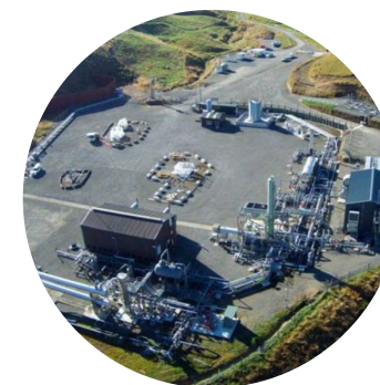
Creating fuel and plant flexibility
