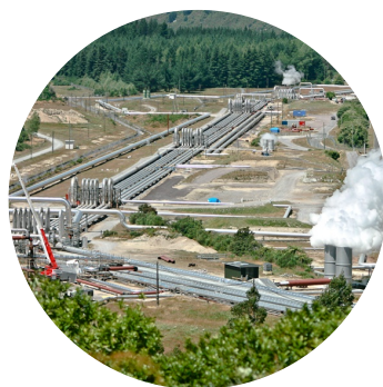
Considering PPA Geothermal
