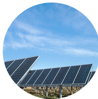
Considering PPA Solar
