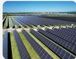
Lauriston Solar Farm
