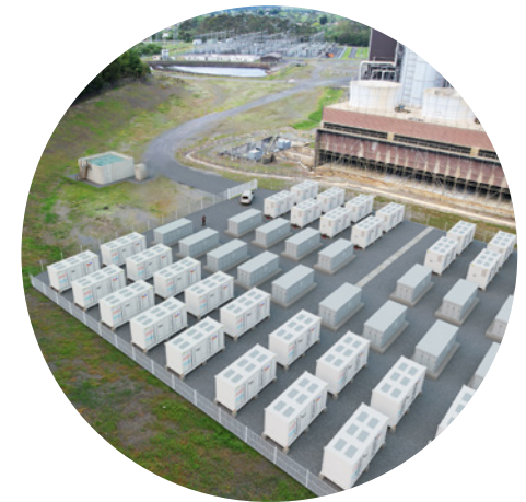
Artist’s impression of the battery installation at Huntly Power Station.
