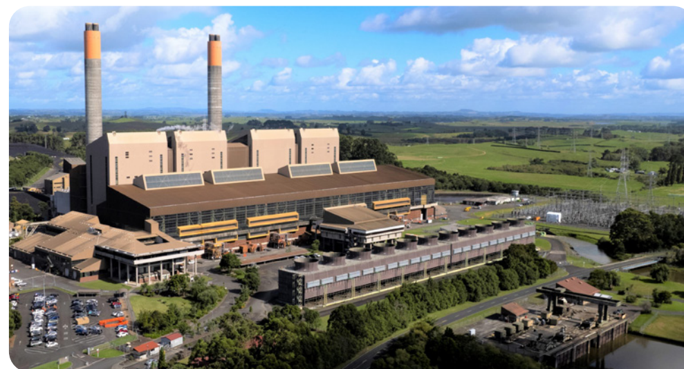
Huntly Power Station
