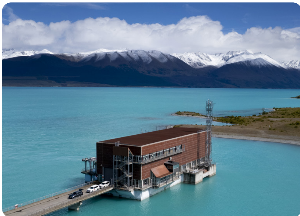
Tekapo B Power Station
