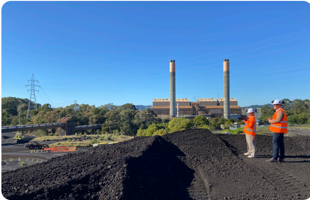
The coal stockpile at Huntly Power Station
