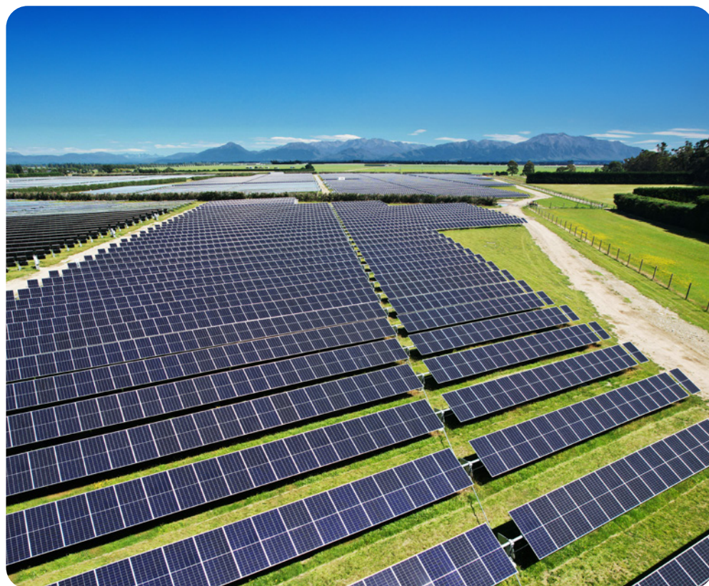
Lauriston Solar Farm
