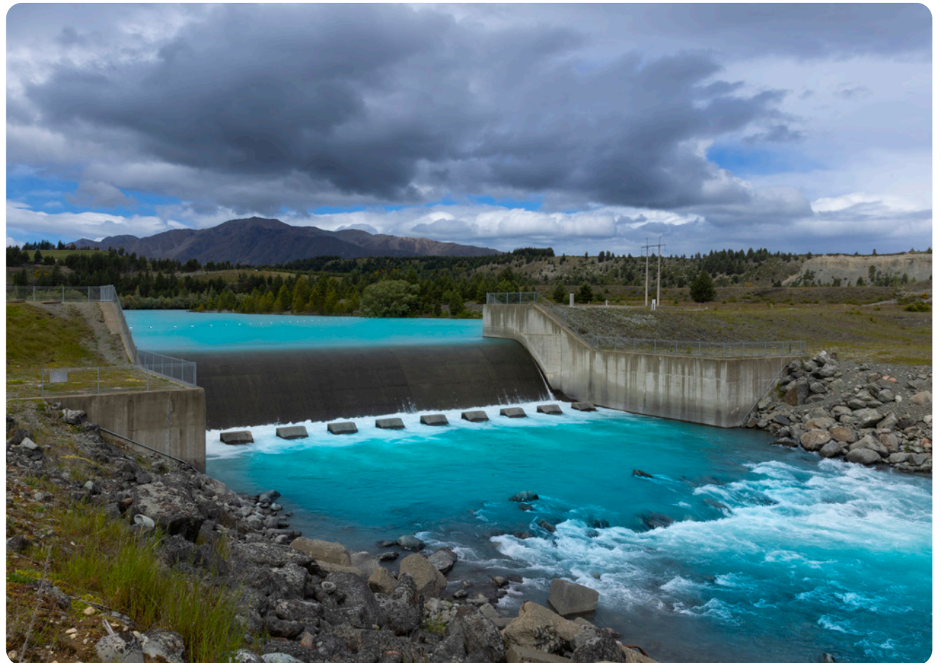
Above: Tekapo A power scheme
